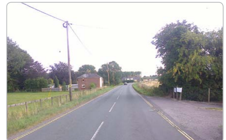
Recommended location of 30mph speed limit - would minimise the visual impact of statutory signage on the landscape. Centre line removal is recommended to help reinforce the change in environment to drivers
