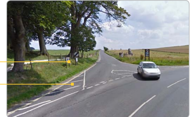
Closure of route reduces or removes need for signing and road markings.
