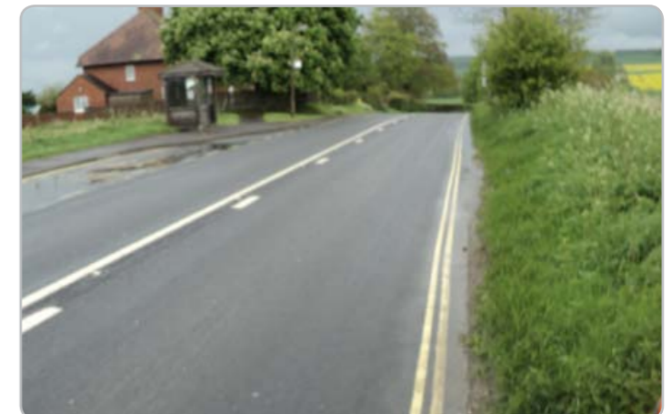
The A4361 between National Trust Car Park and Beckhampton Roundabout
